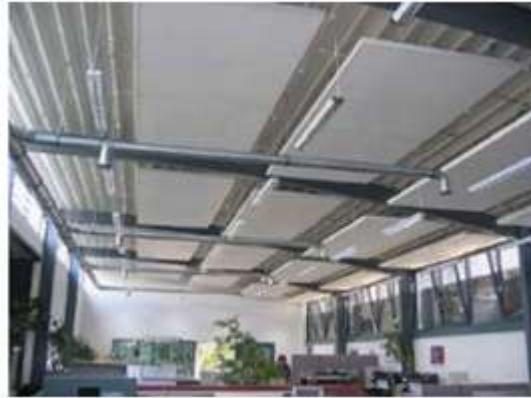
Fig. 18: Sketch of the cooling ceiling with PCM plasterboard circulating of outside cold air under the floor space the PCMs starts discharging and change to solid phase. [43].
