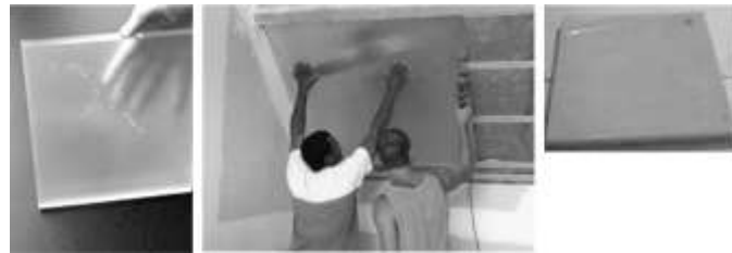
Fig. 12: Left to right: a paraffin-based phase change material (PCM) within a polyester based panel from NovaTherm laboratory. installation of a DuPont Energain panel. Plate PCM
